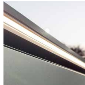
LED Ambiental lighting under the stone worktop
